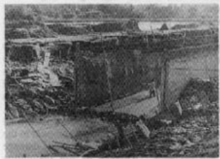
Figure 4 Storm sewer construction while earth filling surrounding natural drainage channel
