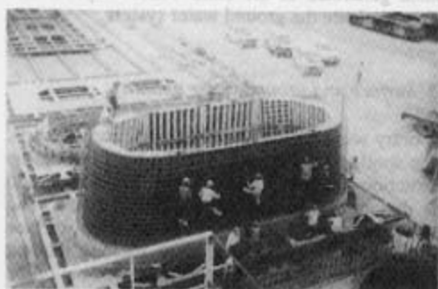
Figure 4 Precast pile cap reinforcement fabrication
