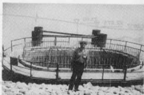
Figure 5 Precast pile cap ready for concreting
