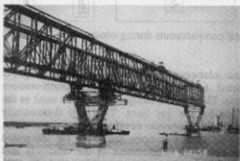
Figure 7 Launching gantry for erection of box girder
