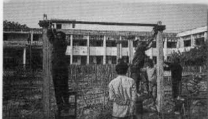
Fixing beam base plate with coupling
