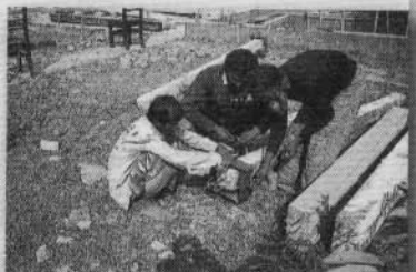
Fixing coupling at pillar top end
