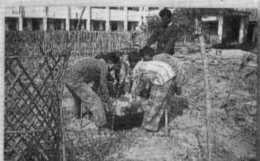
Placing footing base to foundation trench
