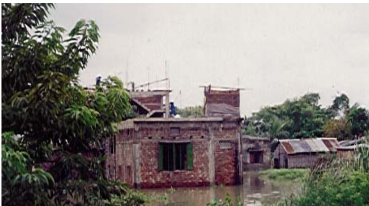
Figure 3: Temporary latrine on roof in flooded area
