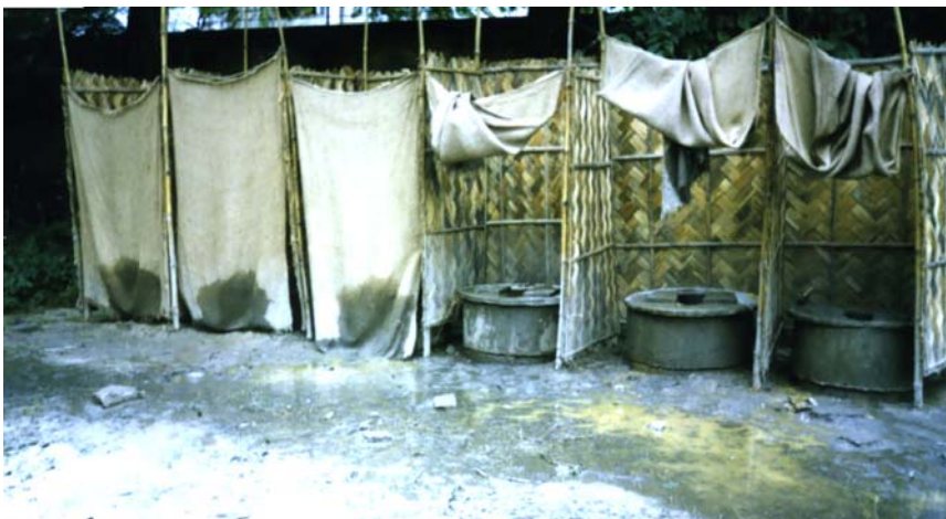
Figure 9: Temporary toilets installed in one shelter
