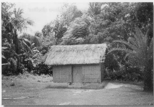
Figure 4 : Thatch-Bamboo shelter
