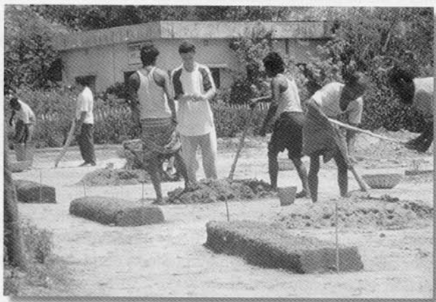
Figure 6 : A practical exercise in mud wall-building
