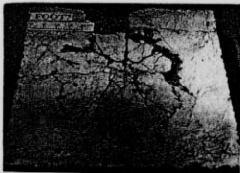
Crack pattern on underside of FOOT1, FOOT4 and FOOT7 tested
