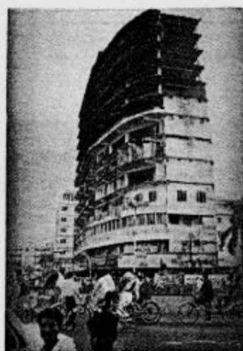
Figure 5. A 13-storey Framed Structure Stands at Heart of City without Occupants It required the concerned authorities quite some time before discovering design faults and stopping construction and occupancy to avert possible disasters.
