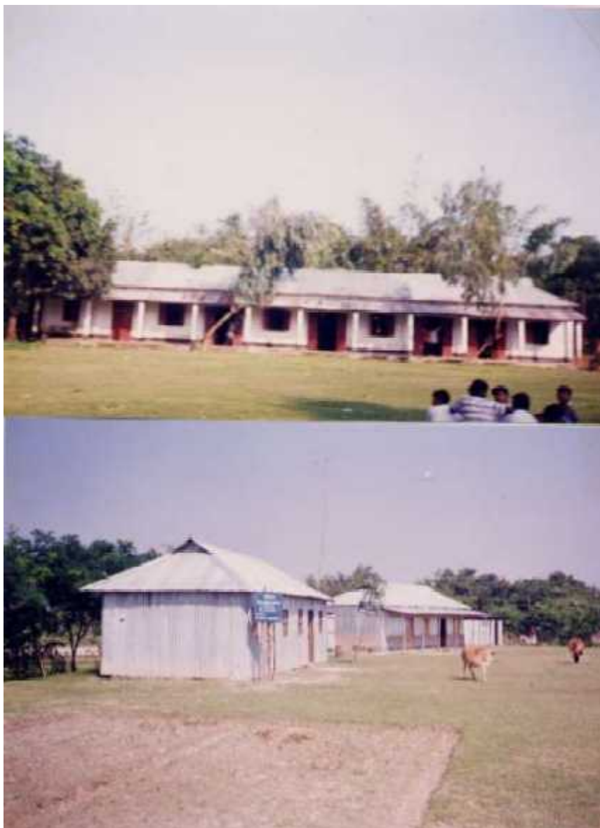
Figure 2: Photograph of Zibika Flood Shelter
