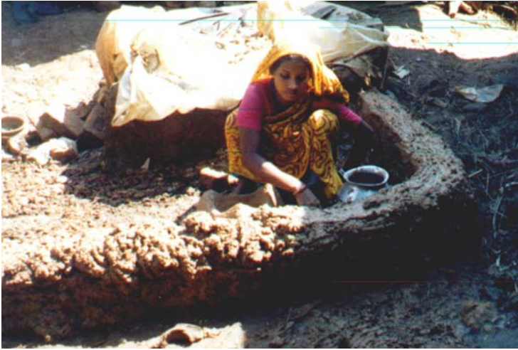
Figure 9: Rebuilding of Vitte washed away by flood
