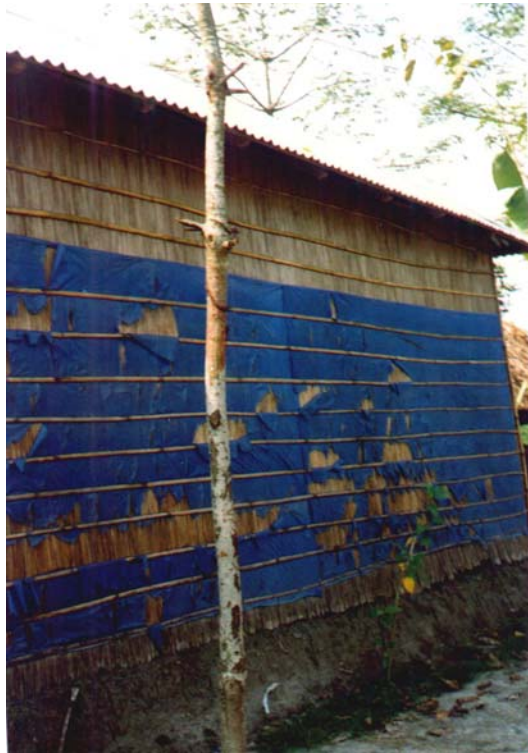
Figure 11: Bera protection using polythene sheet
