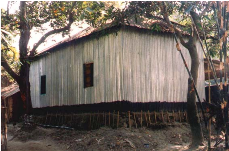
Figure 10: Mud-plinth ( Vitte ) protection using bamboo
