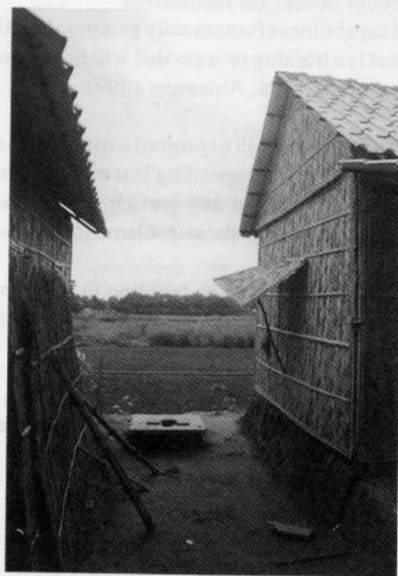
Figure 5 : The position of latrine between houses, causing discomfort to the users. Proshika Palli in Diabari, Manikgonj.
