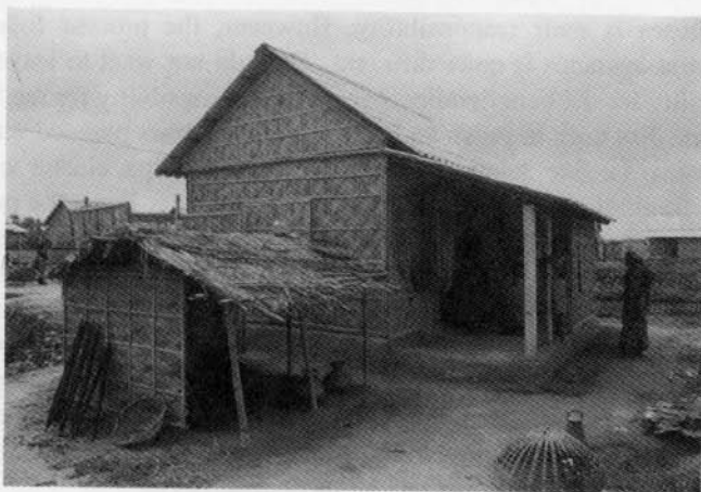
Figure 4 : New kitchen added outside the basic house, Proshika Palli in Diabari, Manikgonj
