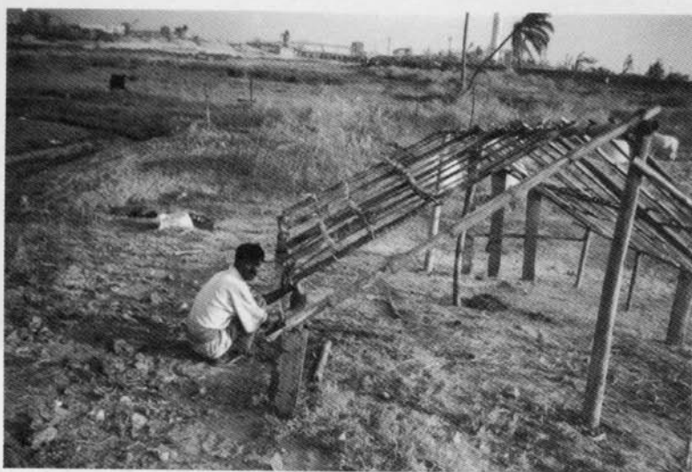
Figure 6 : People affected by the cyclone started construction of their houses again. Mud, thatch and bamboo constitute the primary building materials in the cyclone-affected areas.
