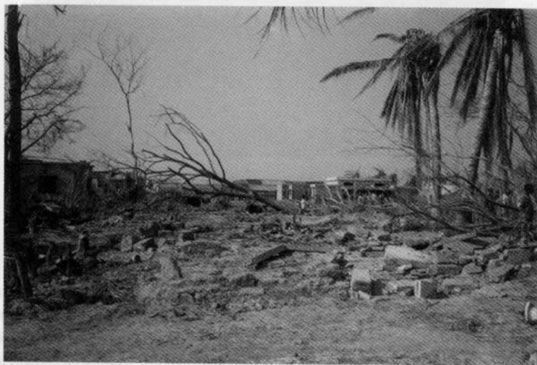
Figure 2 : The houses built by thatch etc. were washed away by the high winds and sea surges. There are no traces left of those houses after the cyclone.
