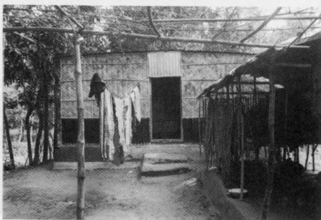
Figs. 6, 7 : Stages of incrementally building the demonstration house
