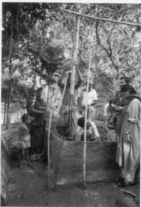
Fig. 4 : Building the demonstration house
